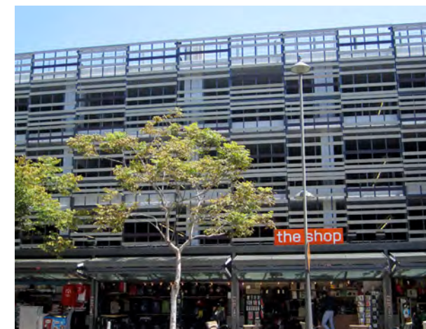
Spaces for temporary galleries and incubator spaces in the City Center Parking Garage
