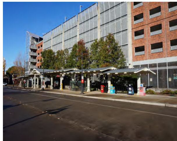
City Center Parking Garage with King County Metro Park-and-Ride spaces on top levels
